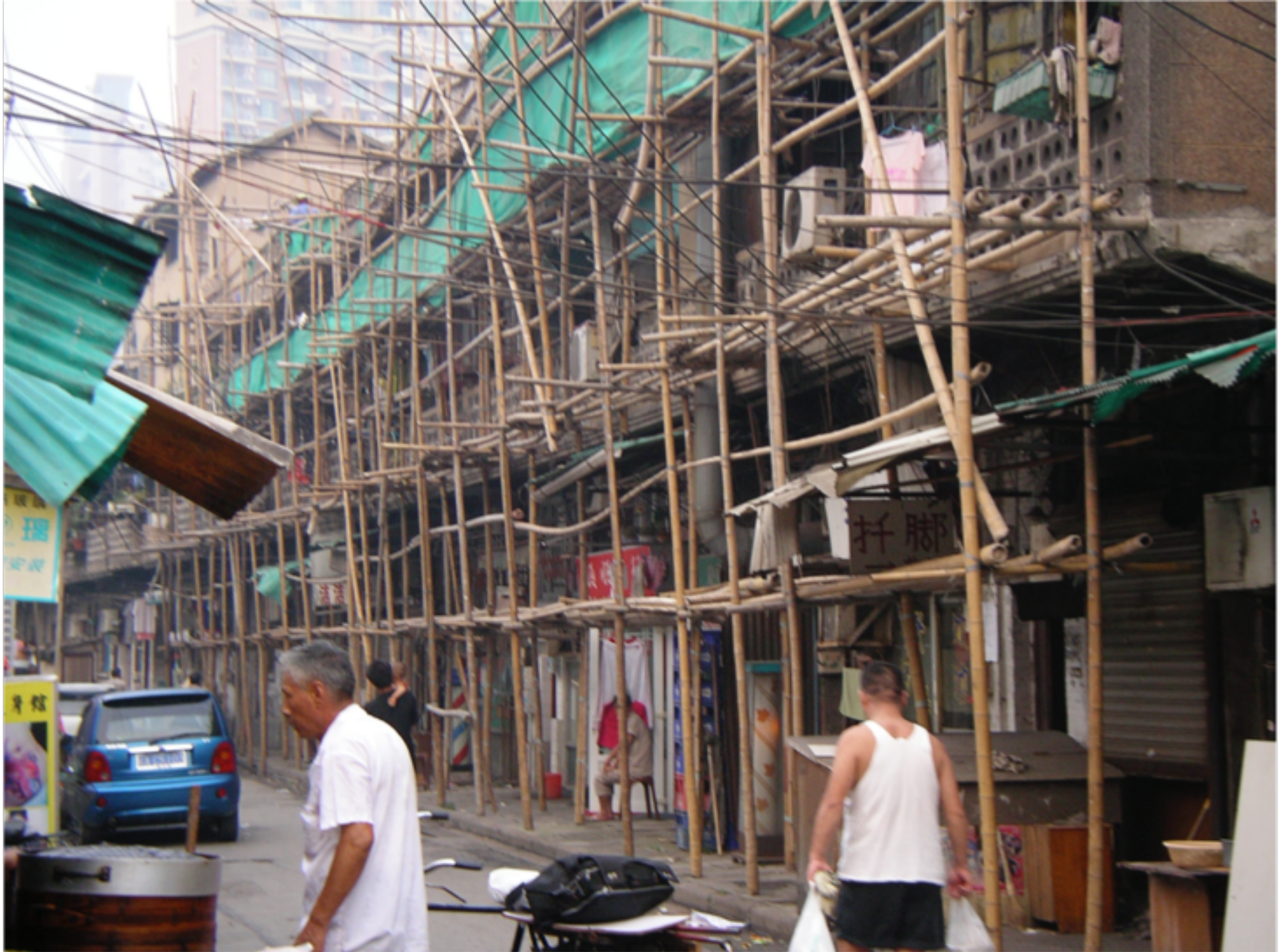
Shanghai, China scaffold (2006)
